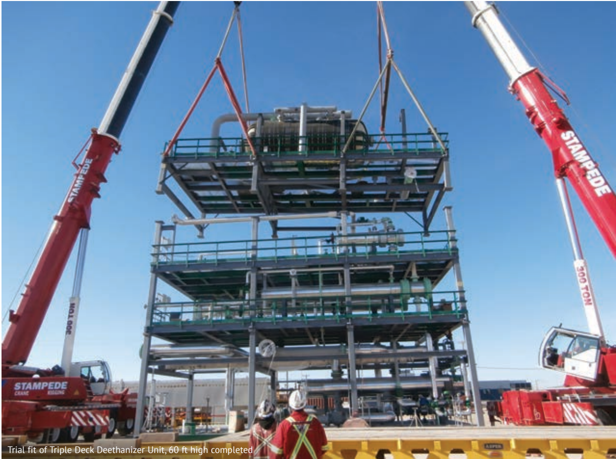
Trial fit of Triple Deck Deethanizer Unit, 60 ft high completed
